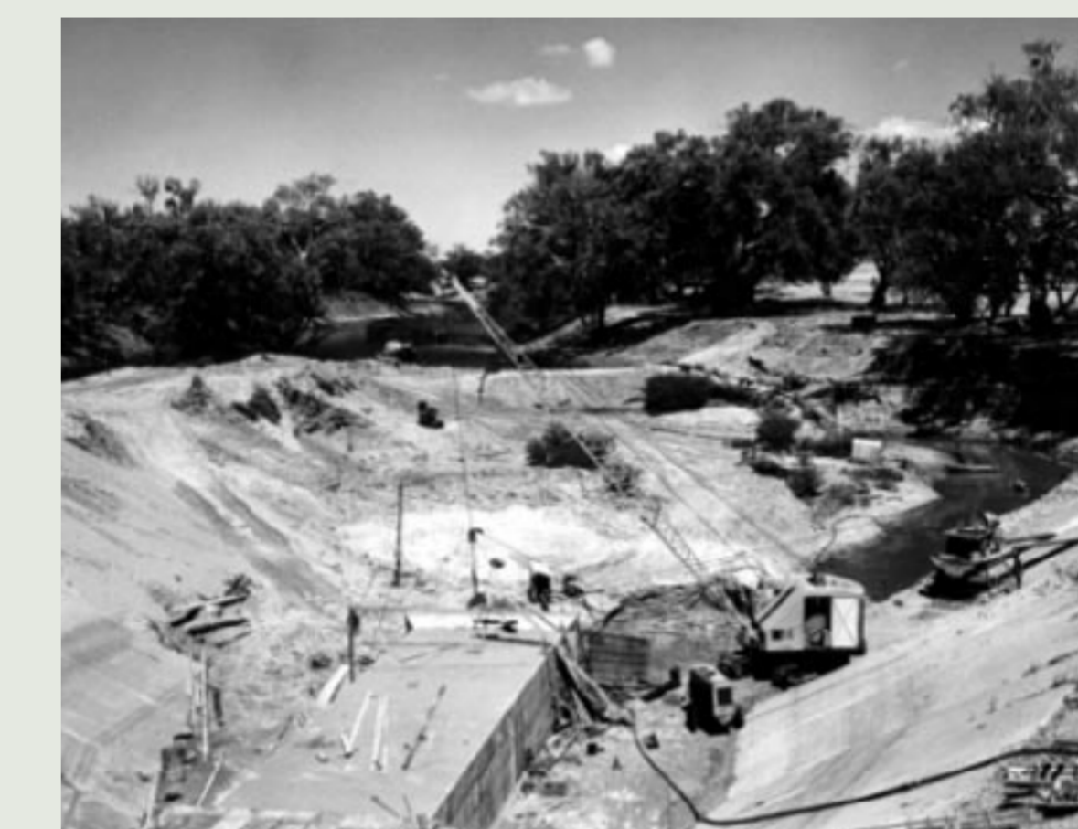
Water Commission pipeline.
