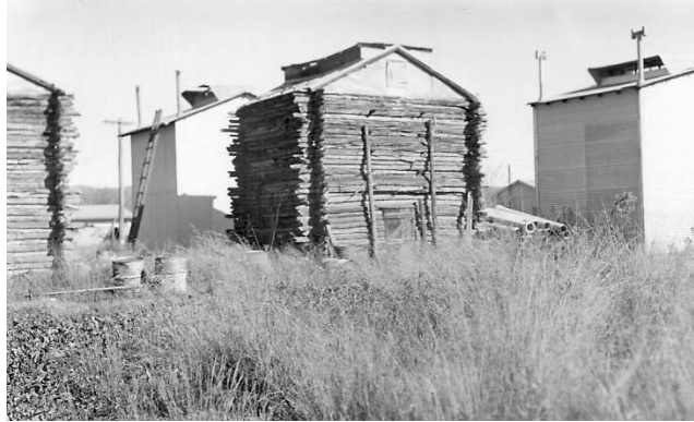
Wooden and cement tobacco barns, Mingoola/Bonshaw area, late 1980s. 40
