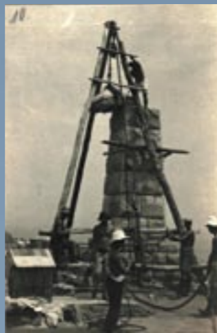
Above: Constructing the stone cairn, c. 1918, photograph, Paul Dubotzki Collection
