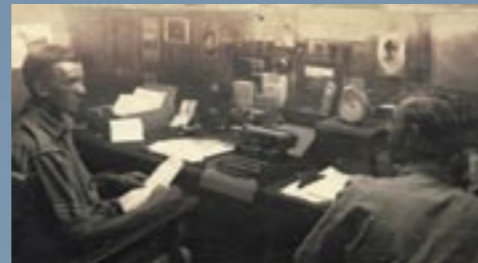
Left: Military Censors at work at Trial Bay, c. 1918, photograph Paul Dubotzki Collection
