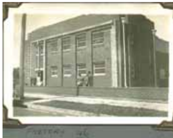
right: L.E. Isaacs Pty Ltd purpose built factory building Gladstone Avenue at the time of its opening in 1946. (photo: Julia McCammon Collection)
